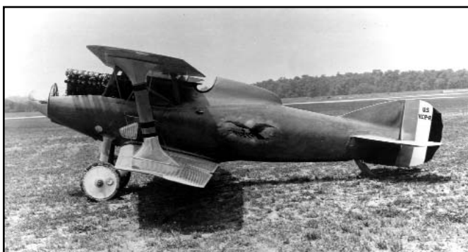
VCP-1 as modified to become VCP-R shown here with the upper engine cowl removed. Author's Collection.
