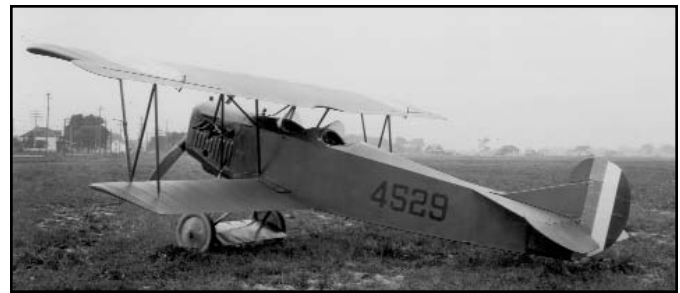
Fokker D-VII No. 4529 loaned to Packard by the Army Air Service for testing. The plane was converted to two-seat configuration by Packard and used for testing 1A-744 and 1A-825 engines. Author's collection.
