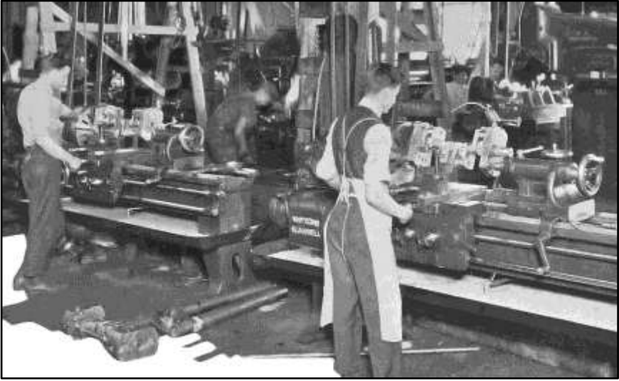
Duesenberg workers machining crankshafts for the King-Bugatti.
