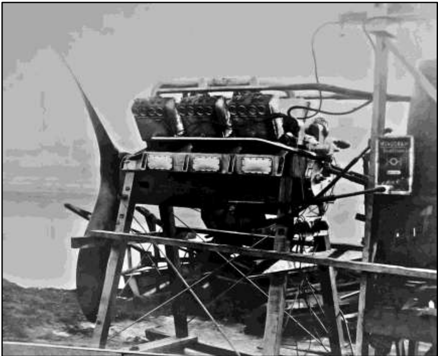
The V-12 ready for a run on a test stand. This appears to be the left side view of the same set-up seen on the opposite page.
