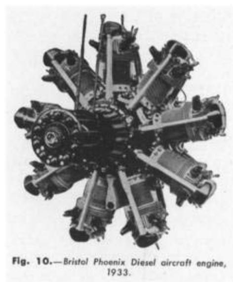
Fig. 10.—Bristol Phoenix Diesel aircraft engine, 1933.
